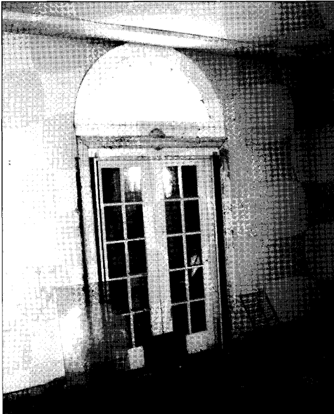
First floor doorway with its fanlight. The fanlights in the Cleaver House admitted light into the entry hall and office.
